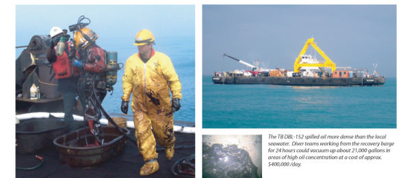
The TB DBL-152 spilled oil more dense than the local seawater. Diver teams working from the recovery barge for 24 hours could recover up to about 21,000 gallons in areas of high oil concentration at a cost of approx. $400,000/day.
