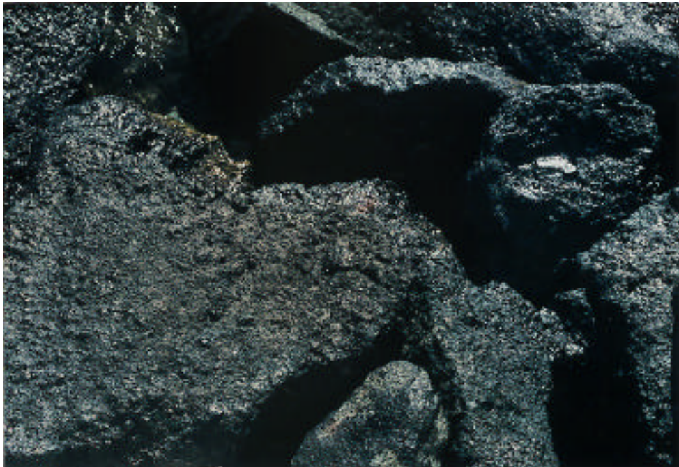
Figure 21B. Plot for high-pressure, hot-water washing alone on rip rap. Pressure and temperature were incrementally increased to 1,200 psi and 175°F. Smooth rock surfaces were cleaned much better than the rough surfaces.
