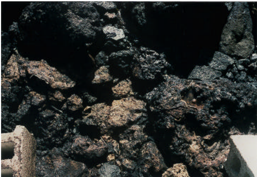
Figure 21D. Plot for the PES-51 cleaner on rip rap with ambient-water-flushing at 1,200 psi.
