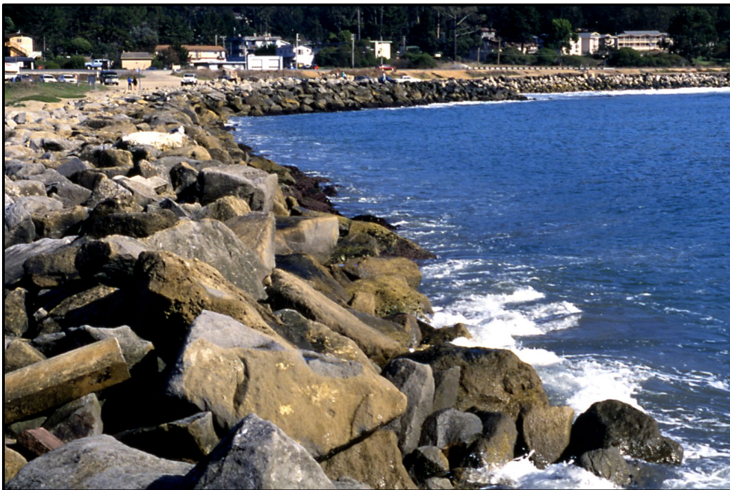
Figure 2.17: Riprap with ESI rank of 6B. Central California.
