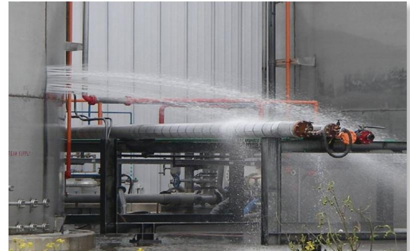
Acid leaking from side of storage tank at chemical facility.
