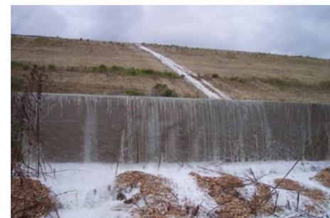
Phosphoric acid spilling from phosphogypsum stack near Houston, TX.
