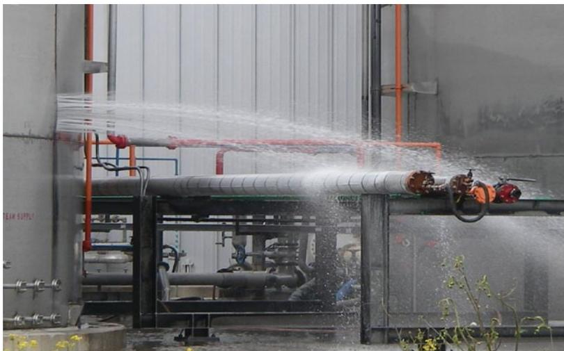
*Acid leaking from side of storage tank at chemical facility.*
